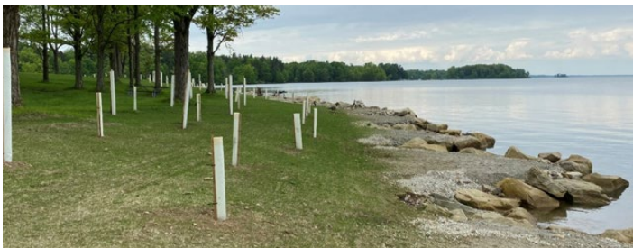
New stone deflectors and tree plantings at the Jamestown Campground at Pymatuning State Park, Crawford County.
